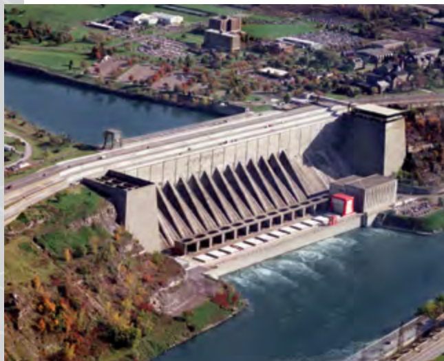
Photo: New York Power Authority
